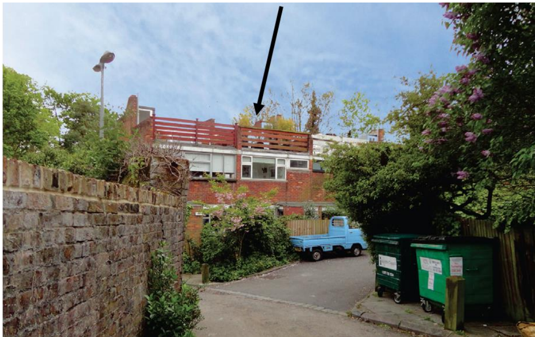
Image 3: Front Elevation of the application site and terrace at 1 – 4 Netherleigh Close
